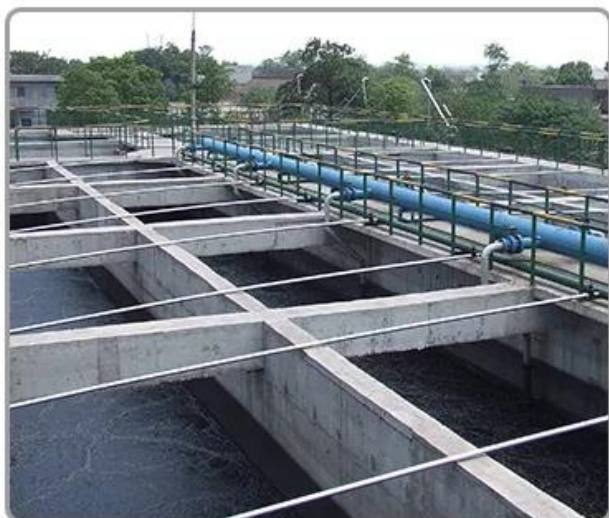
Wastewater treatment plant
