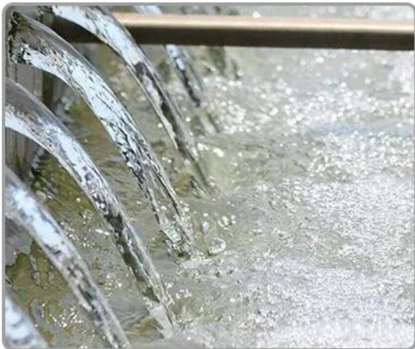
Drinking water plant
